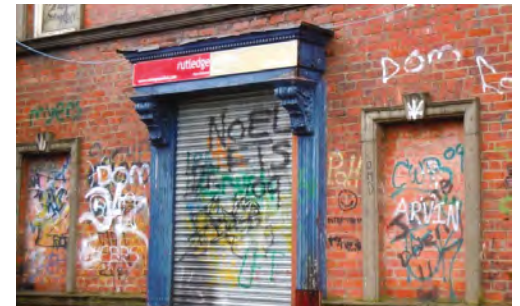
Heavily graffitied building visible from a survey transect
