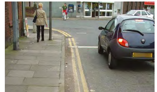
Build-up of detritus forming along the kerbside
